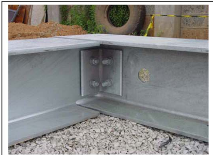
Connection of two corner main beams
