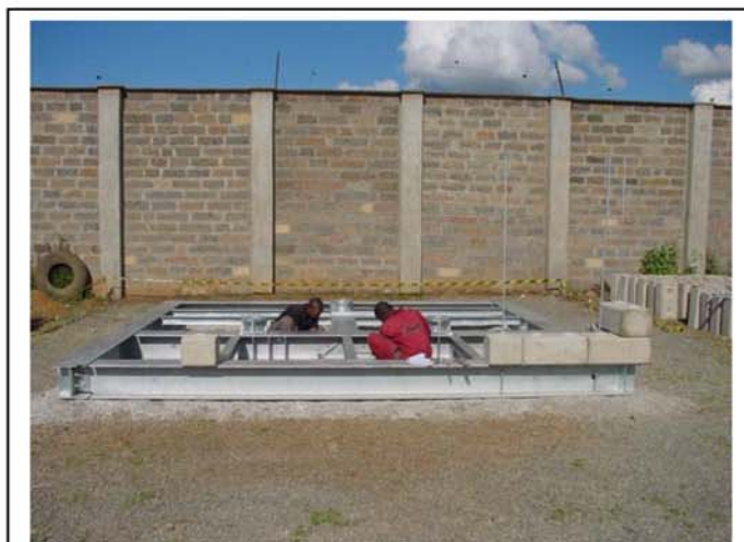
Startup with the placement of the blocks
