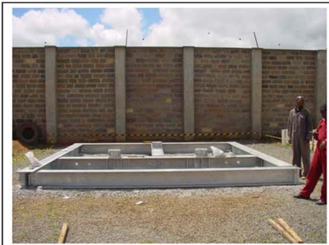
Beam P6 is placed on location. Levels are verified.
