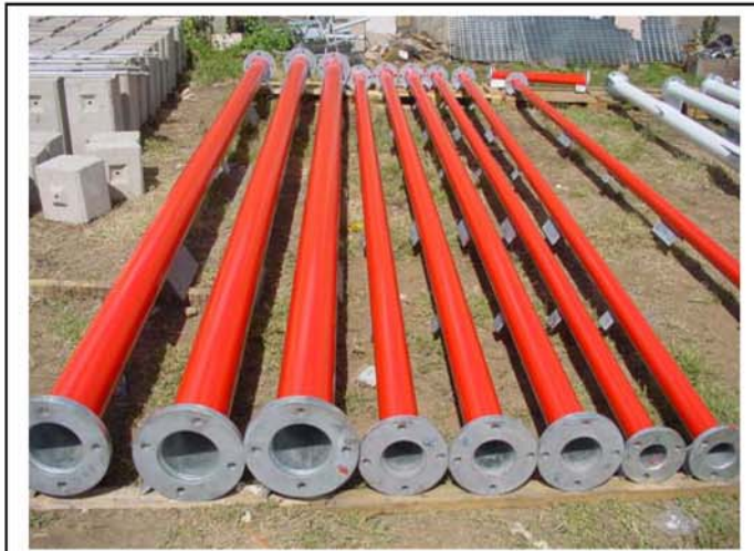
Painting of the first coat of Red paint on the tower
