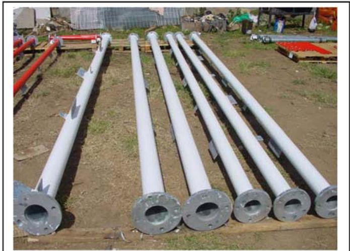
Painting of the first coat of White paint on the tower
