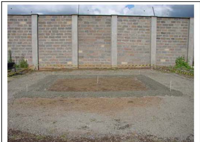
Completed gravel surfacing
