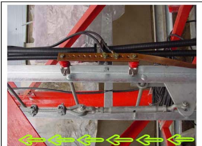
Connection of lower grounding kits.
