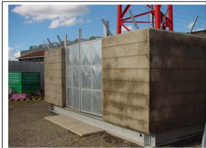
Side view after plastering
