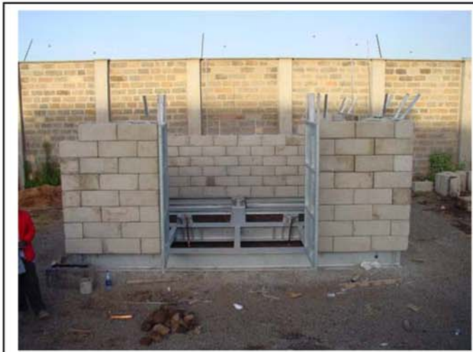
Continuation/Completion of brick wall and Gate Installation
