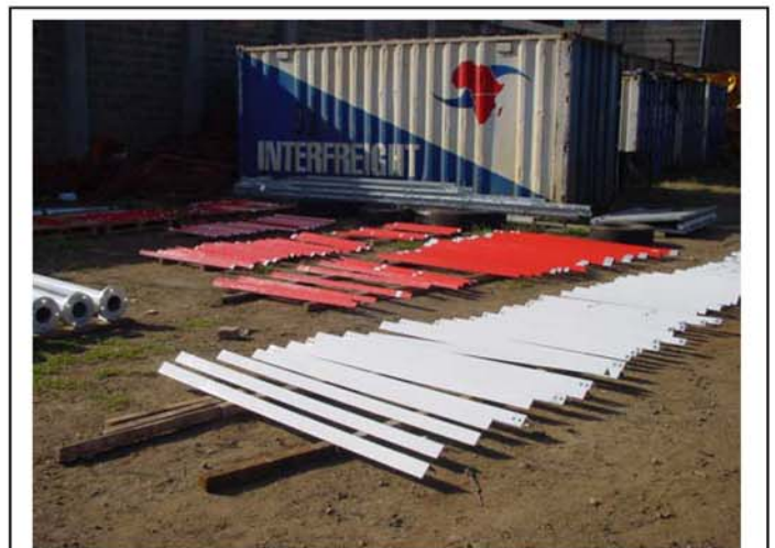
Painting of the Second coat of Red paint on the tower
