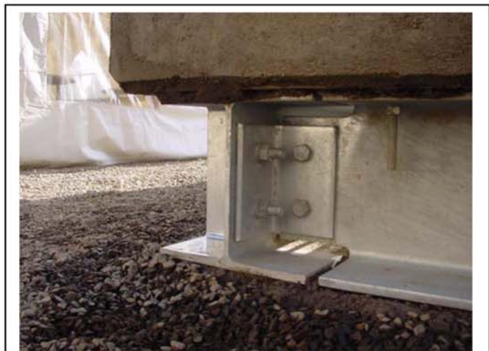
Main beams front connection before plastering
