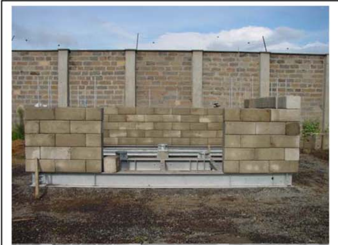
Placement of the blocks – The Rods are continuously inserted to make sure the blocks are in Place
