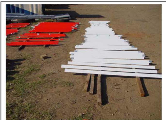
Painting of the Second coat of White paint on the tower
