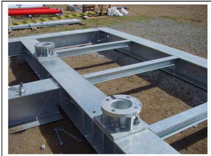
Right side of the complete steel structure
