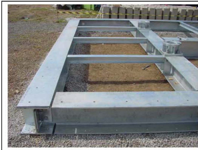
Left side of the complete steel structure
