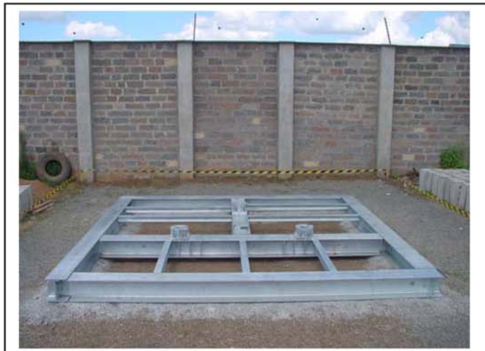
Secondary Beams are also installed. Steel structure is complete
