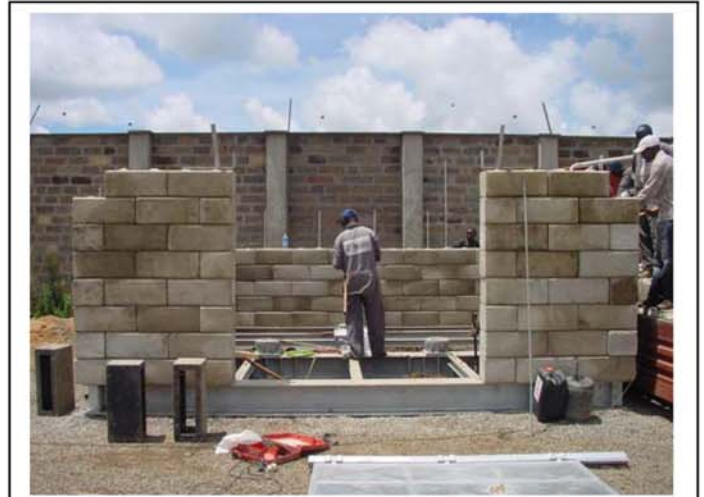
Placement of the blocks – The Rods are continuously inserted to make sure the blocks are in Place
