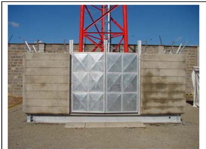
Front view after plastering
