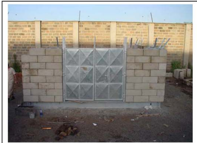
Continuation/Completion of brick wall and Gate Installation
