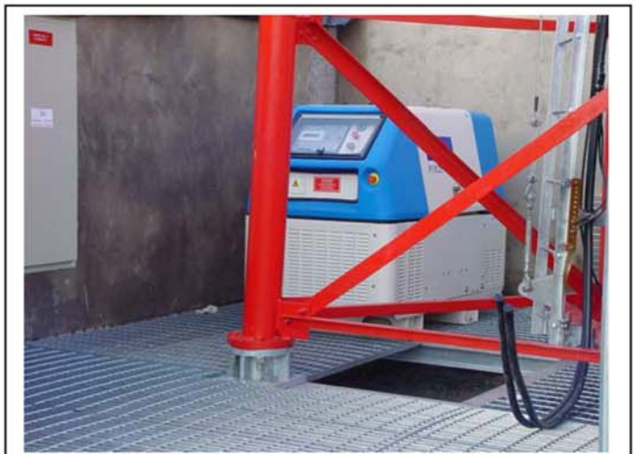
Generator and exhaust pipe installation
