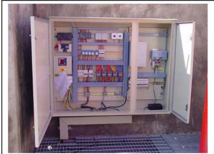
Installation of the Electrical cabinet
