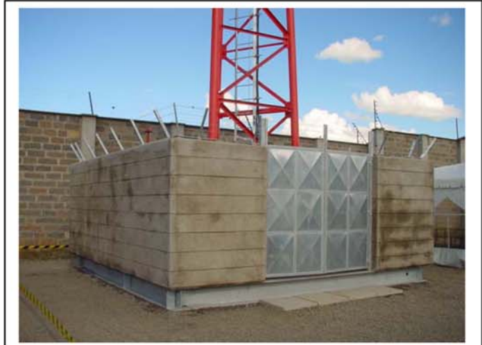
Side view after plastering
