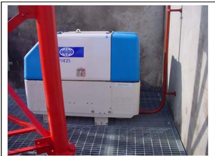
Generator and exhaust pipe installation
