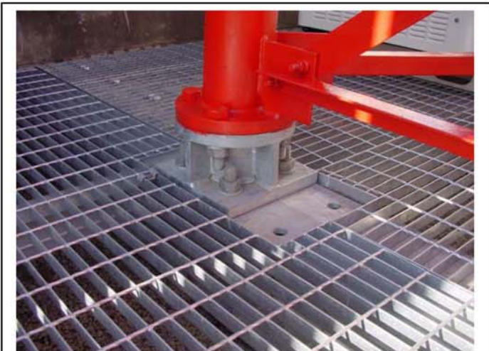
Installation of the Grating
