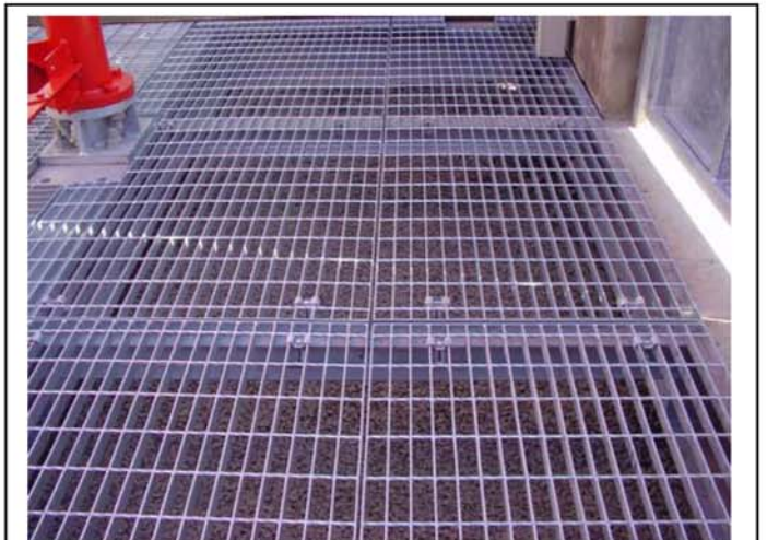
Installation of the Grating
