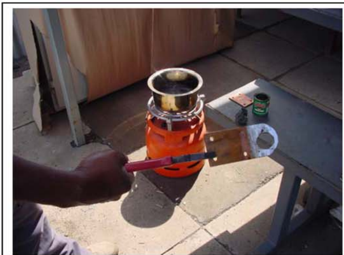
Connection plate after Tinning
