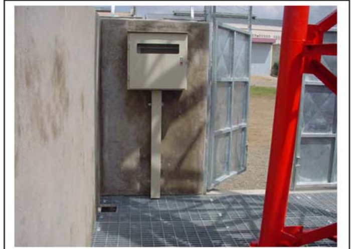
Installation of the energy meter box.
