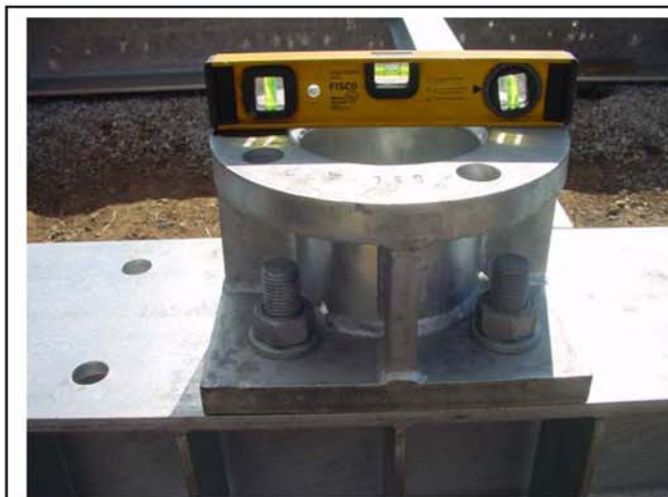
It is essential for all the connection plates to be leveled
