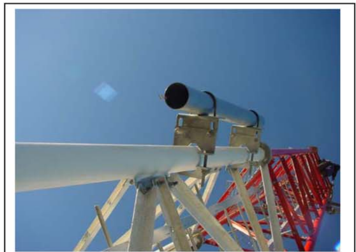
Installation of one MW bracket and two antenna poles
